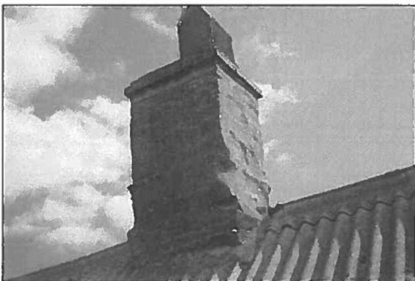
Chimney is sealed with no gaps
